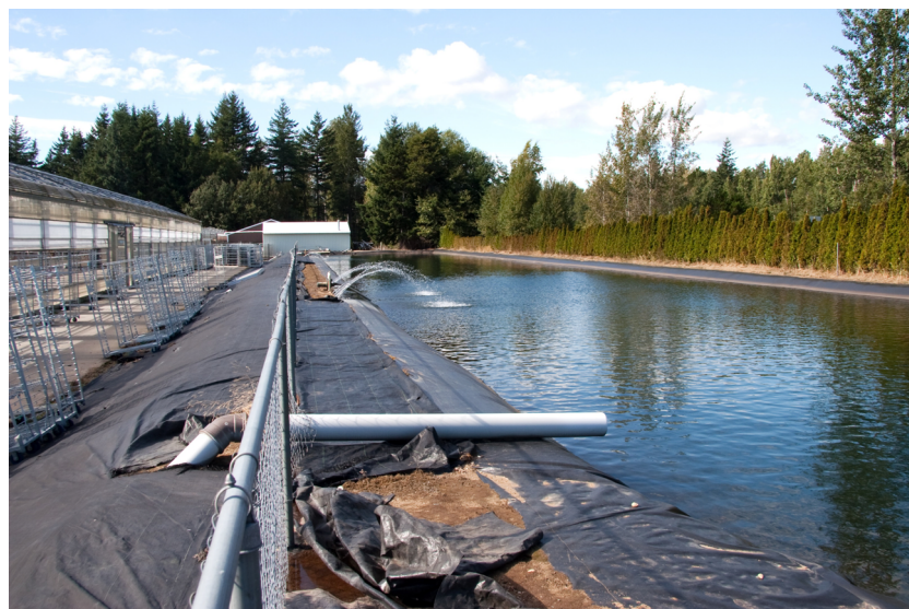
Fig. 2. A fully lined levee pond directly adjacent to a large commercial greenhouse serves as an excellent rainwater harvesting collection basin.
