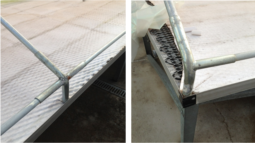
Fig. 2. Conduit electrical metallic tubing connectors used for the construction of the plastic tent.
