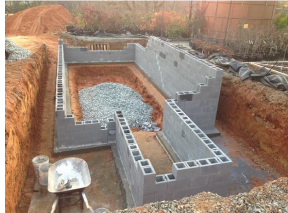
Figure 2. (A) Pit greenhouse is a structure that is earth sheltered, (B) Once level footings are in place, 8-in. concrete blocks are stacked dry without mortar joints.
