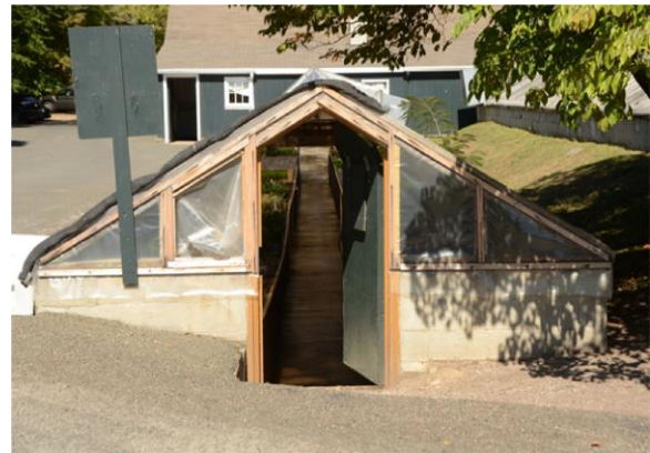
Figure 1. Earth shelter structure at Summer Hill Nursery.
