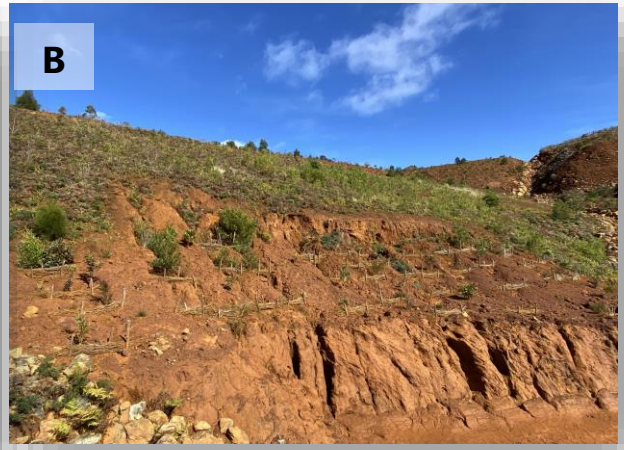
Figure 2. (A) Planting behind wooden windbreakers on sites where strong prevailing winds occur - (B) Planting behind fascines (or dead wood bundles), a technique used on slopes to reduce erosion.
