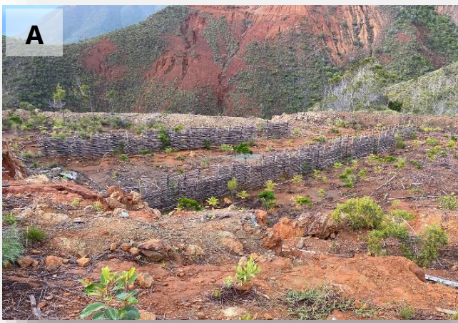
Figure 2. (A) Planting behind wooden windbreakers on sites where strong prevailing winds occur - (B) Planting behind fascines (or dead wood bundles), a technique used on slopes to reduce erosion.
