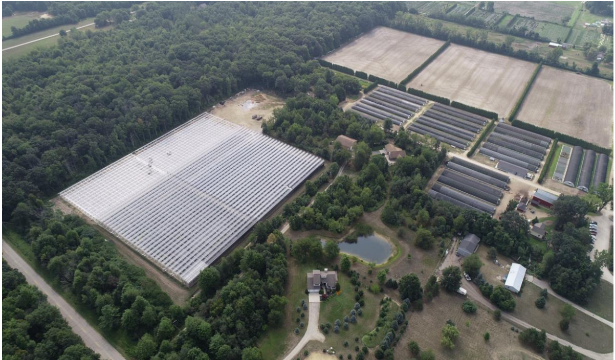
Figure 10. Aerial photograph of Spring Meadow Nursery's 10-acre Research and Development facility.
