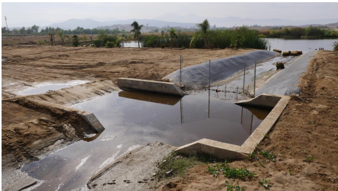
Figure 3. Sediment forebay designed for easy clean out.
