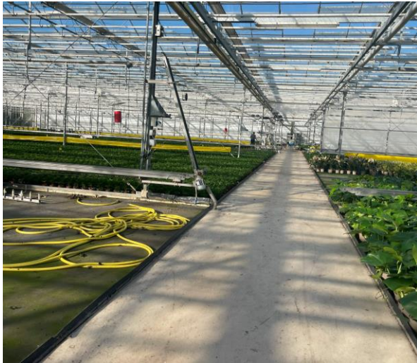
Figure 2. Floor irrigation and belt system and Hills Nursery.
