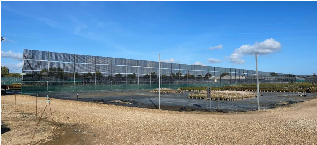
Figure 3. Wind barrier at Walberton.
